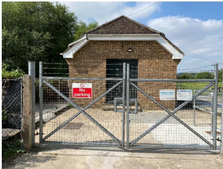
Photo 2: Hanging Langford pumping station, pumping flow to Great Barford WRC for treatment, and overflowing to the reedbed located on Langford Lakes Nature Reserve 'Hanging Langford reedbed'
