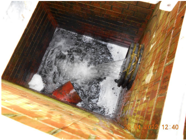
Photo 3: Discharging outfall from the reedbed at Hanging Langford on 28/01/2022.
