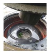
Mullens Pond WPS Wear on impellers No critical spares (lesson learned) Experiments with various pumps and impellers Aim for better pass forward to minimise interventions
